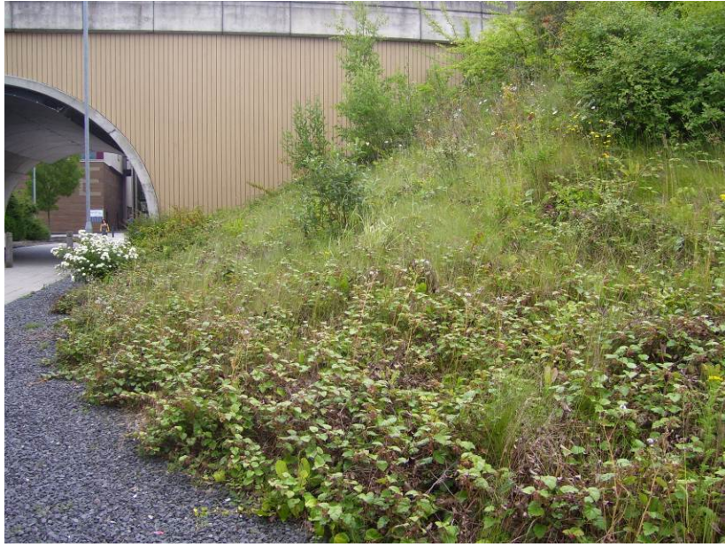
Photograph 3: landscaping shrubs and rough grass on embankment up to Brayford Way
