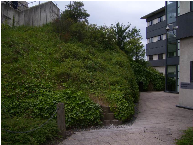
Photograph 5: landscaping shrubs and rough grass on embankment up to Brayford Way
