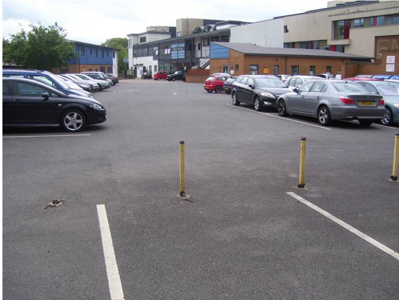
Photograph 1: general view of the car park
