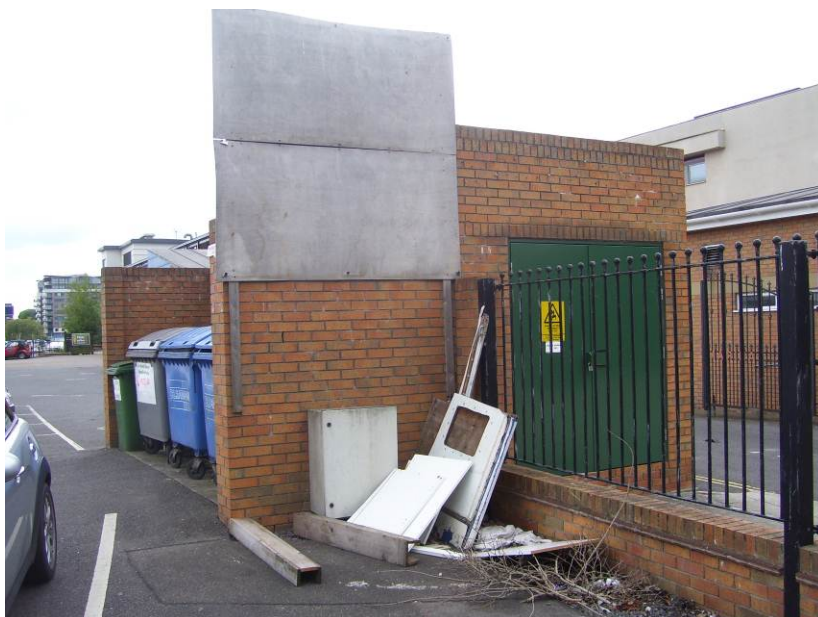
Photograph 2: bin store and sub-station buildings
