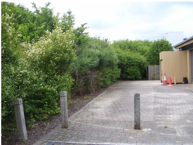
Photograph 2: landscaping shrubs behind electricity sub-station
